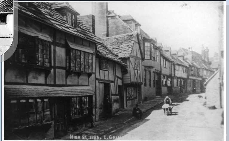
Middle Row - Looking West
