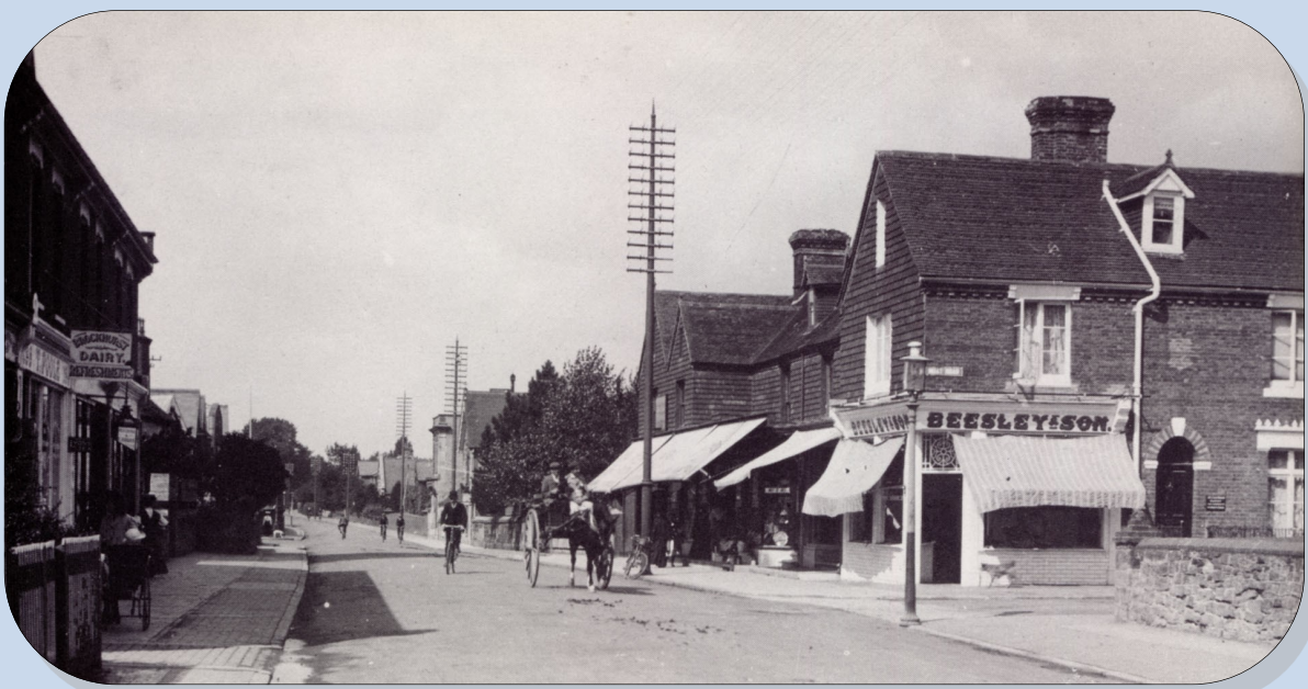
London Road. Looking North-1910
