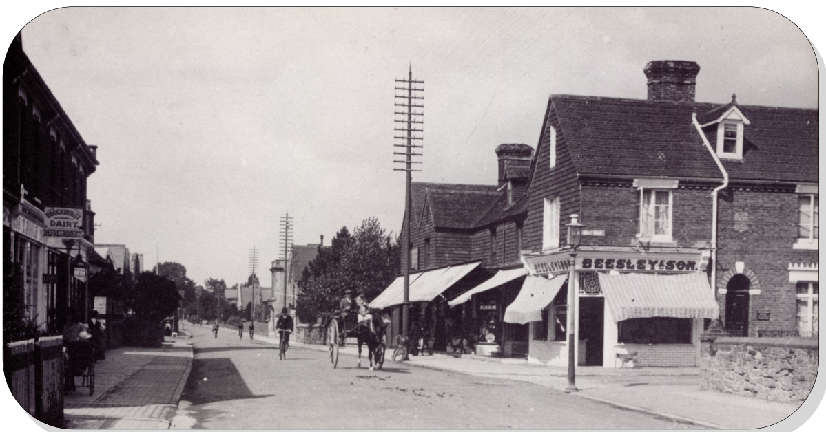
London Road. Looking North-1910
