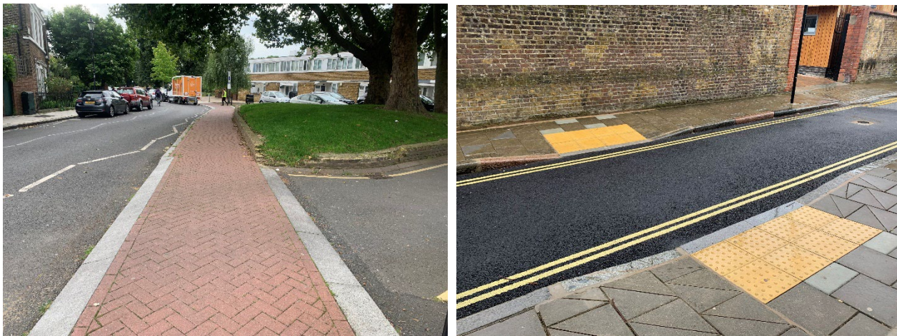
Figure 7-1: Continuous footway provision (Left – Claylands Road) and Dropped kerb with tactile paving (Right – Sans Walk)
