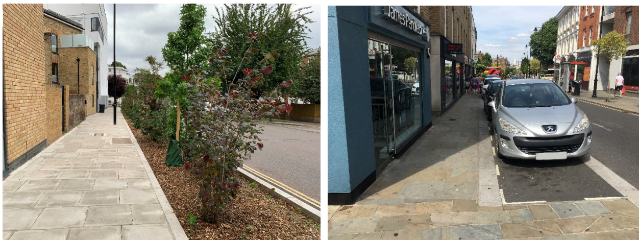
Figure 7-4: Example of clear footway space incorporating SUDs (Left – Crossway) and Recessed loading pads enable footway widening in constrained streetscapes (right – Clapham Old Town)
