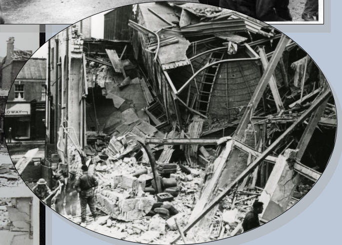
Bomb damage to London Road
