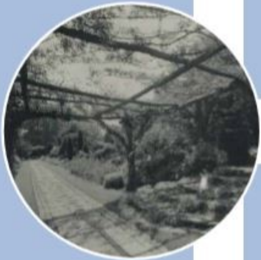
The Lower Terrace at East Court looking west
