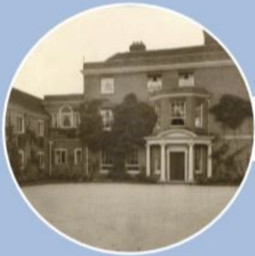
Main entrance to East Court (used to be the back door!)
