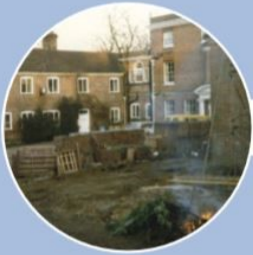
Remodeling to make way for The Meridian Hall
