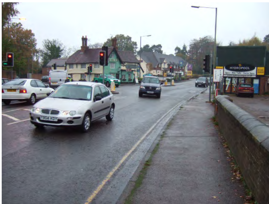
Figure 8. A22 Looking North with Bridge over Stream to Left
